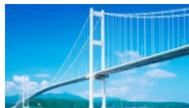
● 桥梁位移监测 Bridge displacement monitoring
